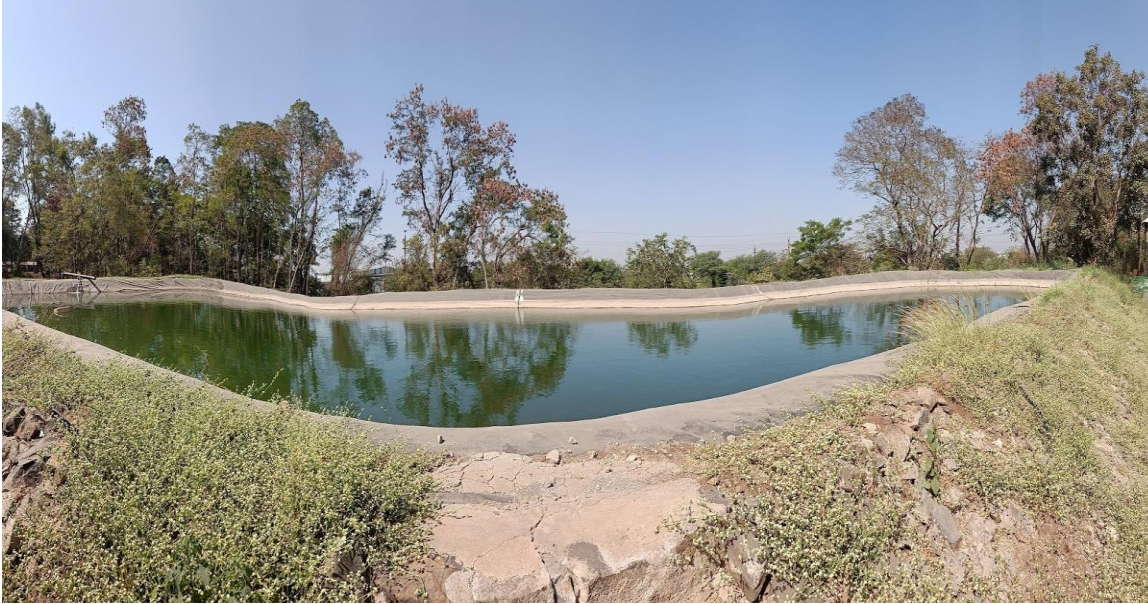
Pond Capacity - 6 Million Litres
