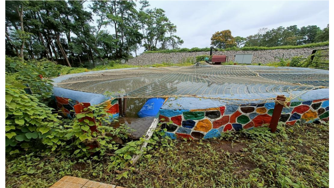
UG open Tank Capacity - 1 Million Litres
