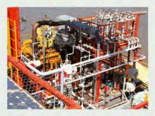
Gas Engine Driven Reciprocating Gas Compressor Package for an Unmanned Off-shore Platform
